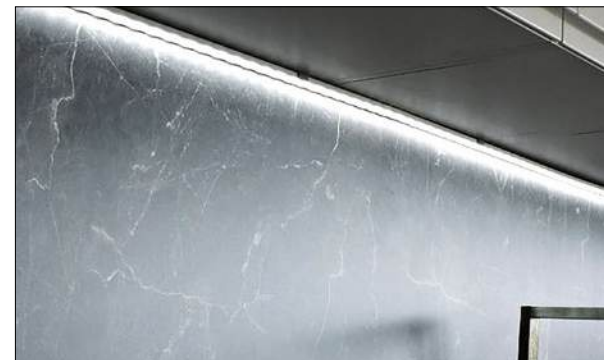
Wall Unit Strip Lights
